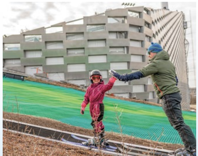
Three Moving Carpets for inner-city skiing in Copenhagen (Denmark)
