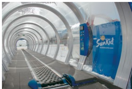
Operation terminal inside the gallery
